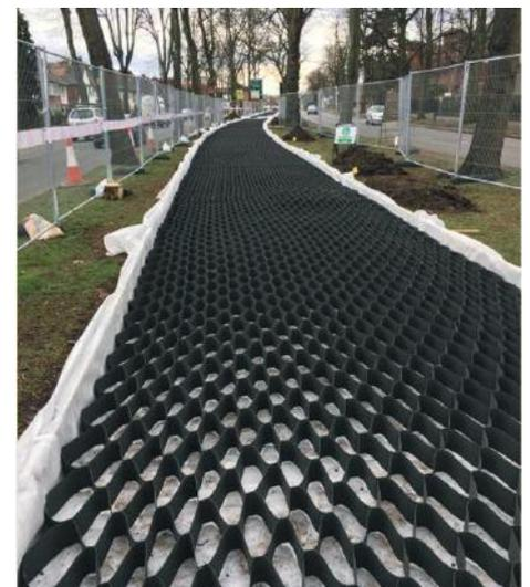
8. Fill the Terram Geocell with a clean, open graded angular aggregate (5mm - 45mm) working towards the tree from the furthest point away and using the filled Terram Geocell as a platform. (Single sized, rounded aggregate or DoT Type 1 should not be used). Do not roll the surface, a light vibratory compaction plate may be permitted to settle the stone into the cells; seek advice from the specifier or Arboricultural Officer. Do not contaminate the filled cells with site debris, soil or mud.
