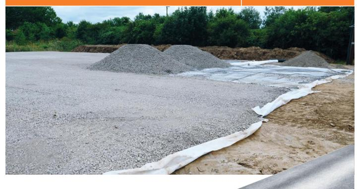
Non-woven geotextile manufactured from UV stabilised, high tenacity, virgin polypropylene fibres that have been both mechanically and thermally bonded to provide a highly permeable yet durable separation and filtration layer.
